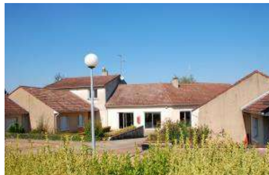
Foyer Soleil , logements CCAS Bouloire 31 places
